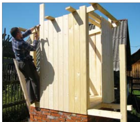
fig. 6: Offsite-Construction of the frame for the toilet room walls from wood (left), covering walls with 2 cm wooden slats (right)
