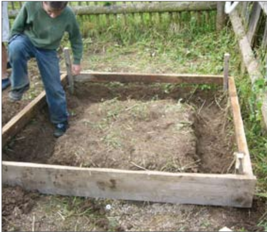
fig. 3: Floor of faeces chambers from concrete: formwork (left), finished (right)
