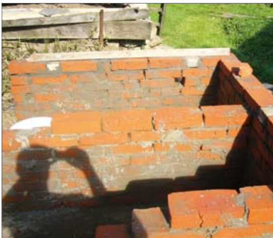
fig. 4: Construction of the faeces chamber outside walls from bricks (left), hole for urine piping (right)
