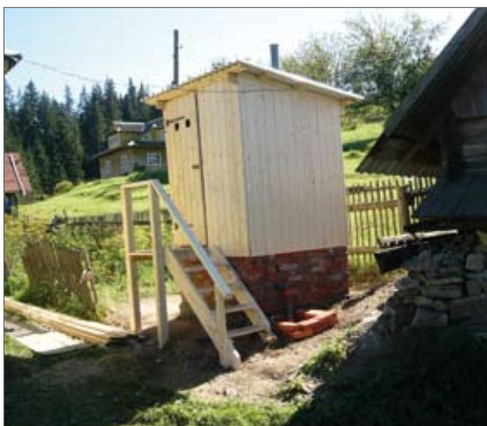
fig. 1: Dry Double chamber UD-Toilet: outside view (left) and inside view (right)
