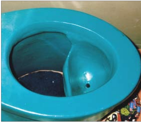
fig. 8: UD-seat riser (left)* and UD-squatting pan (right)
