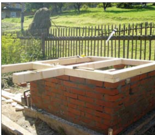
fig. 5: Frame for floor of toilet room (left) and cutting hole for seat riser (right)
