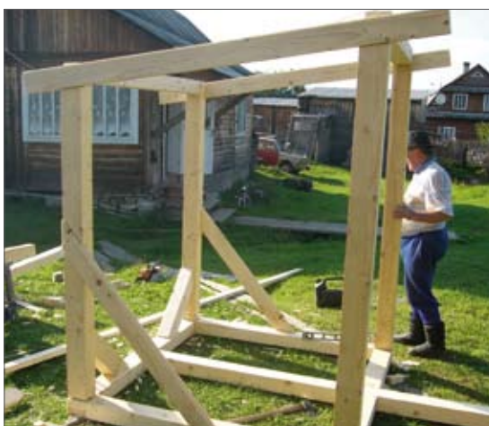
fig. 6: Offsite-Construction of the frame for the toilet room walls from wood (left), covering walls with 2 cm wooden slats (right)
