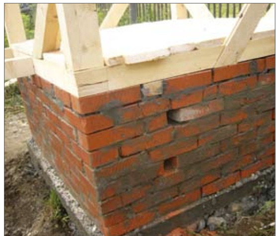
fig. 4: Construction of the faeces chamber outside walls from bricks (left), hole for urine piping (right)
