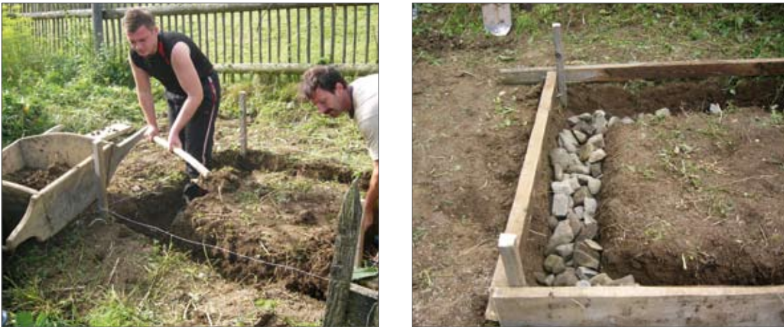
fig. 2: Excavation for round foundation (left) and filling with stones (right)
