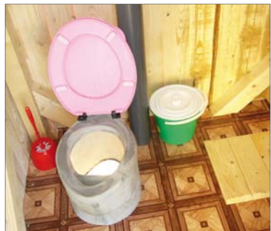
fig. 1: Dry Double chamber UD-Toilet: outside view (left) and inside view (right)
